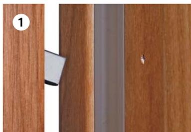
1 After the installation of the lock and the throw of the hook, by softly pushing the door against the jamb it is possible to centre the striker.
