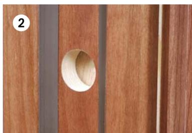
2 The striker installation has never been so simple: it just takes a milling of  $\varnothing 25$  mm and a drill. Jigs are not required.
